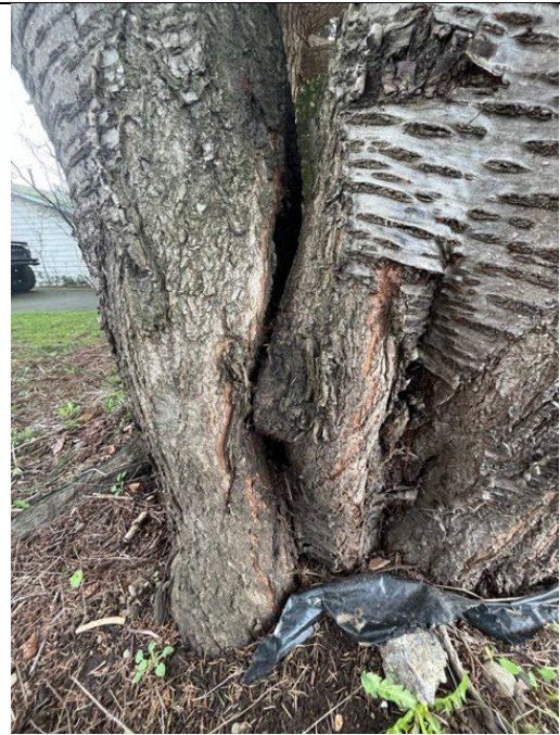
Photo 8. Close-up view of base of Cherry #523/7642 with northern stem (left) noted splitting from the southern stems. North stem assessed to be a high risk, only it requires pruning/removal.
