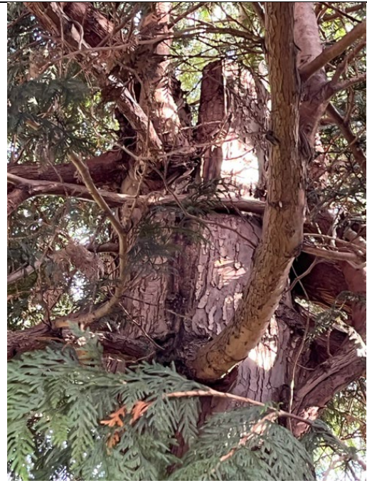
Photo 14. Closeup view of offsite Cedar 3 topped with multiple tops weakly attached to a cracked dead top.
