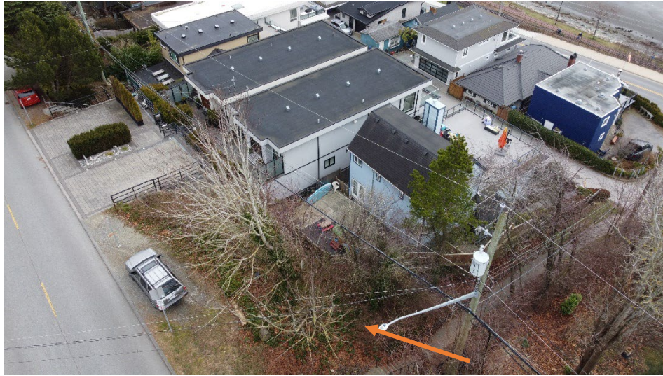
Frontage along Victoria St – corner cut identified
