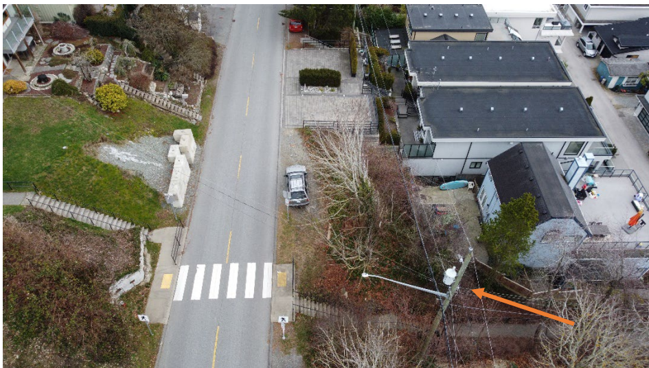
Frontage along Victoria St – corner cut identified
