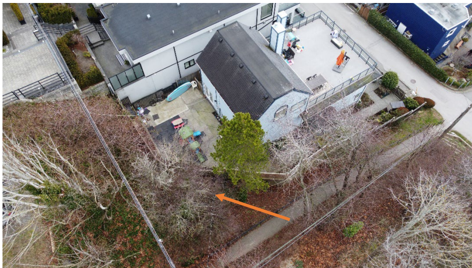
Frontage along Victoria St – corner cut identified
