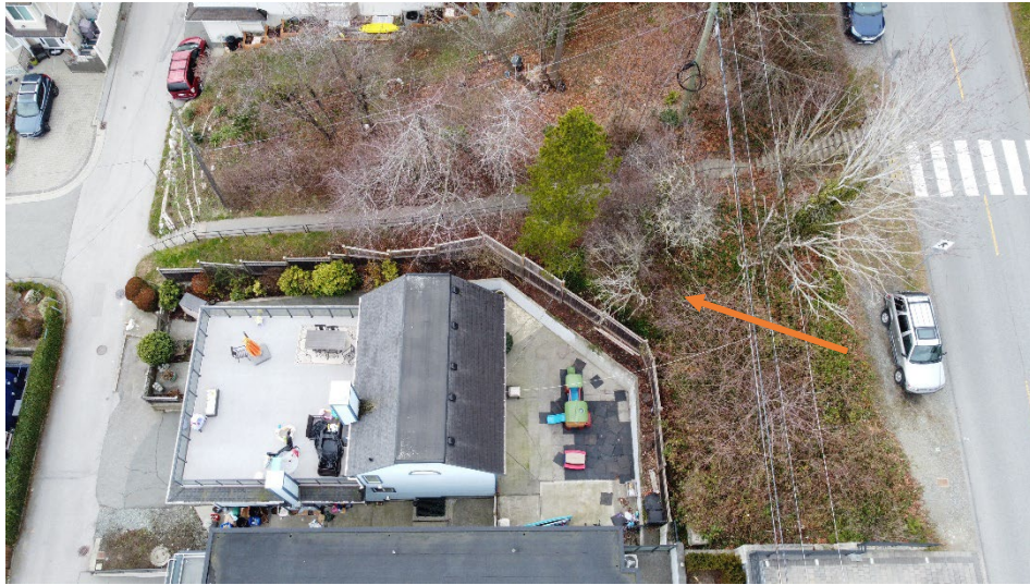
Frontage along Victoria St – corner cut identified
