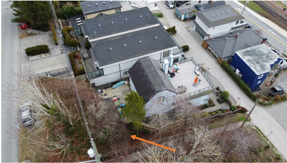
Frontage along Victoria St – corner cut identified
