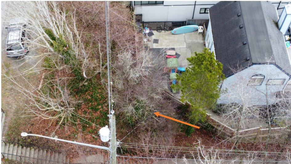
Frontage along Victoria St – corner cut identified
