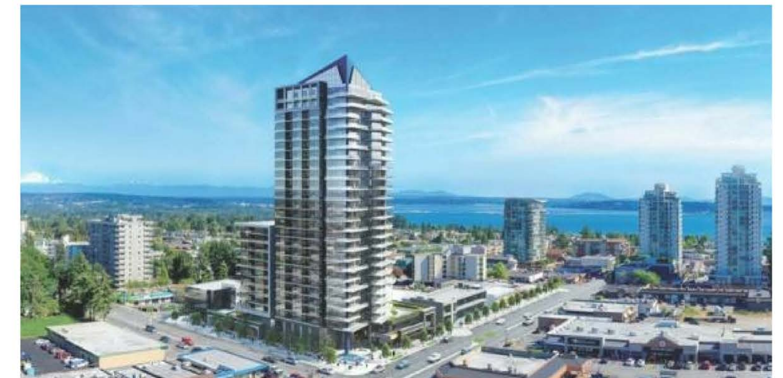
1588 JOHNSTON ST. (CONTINUING CONSTRUCTION)
