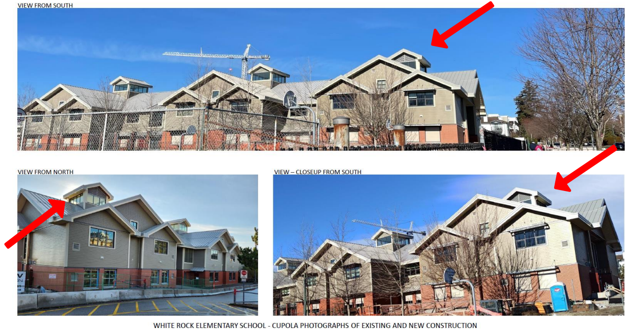
Figure 4 – Photos illustrating completed cupola construction and existing school
