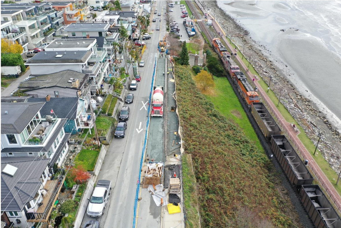
Photo 2: Looking eastward from above top of Hump
