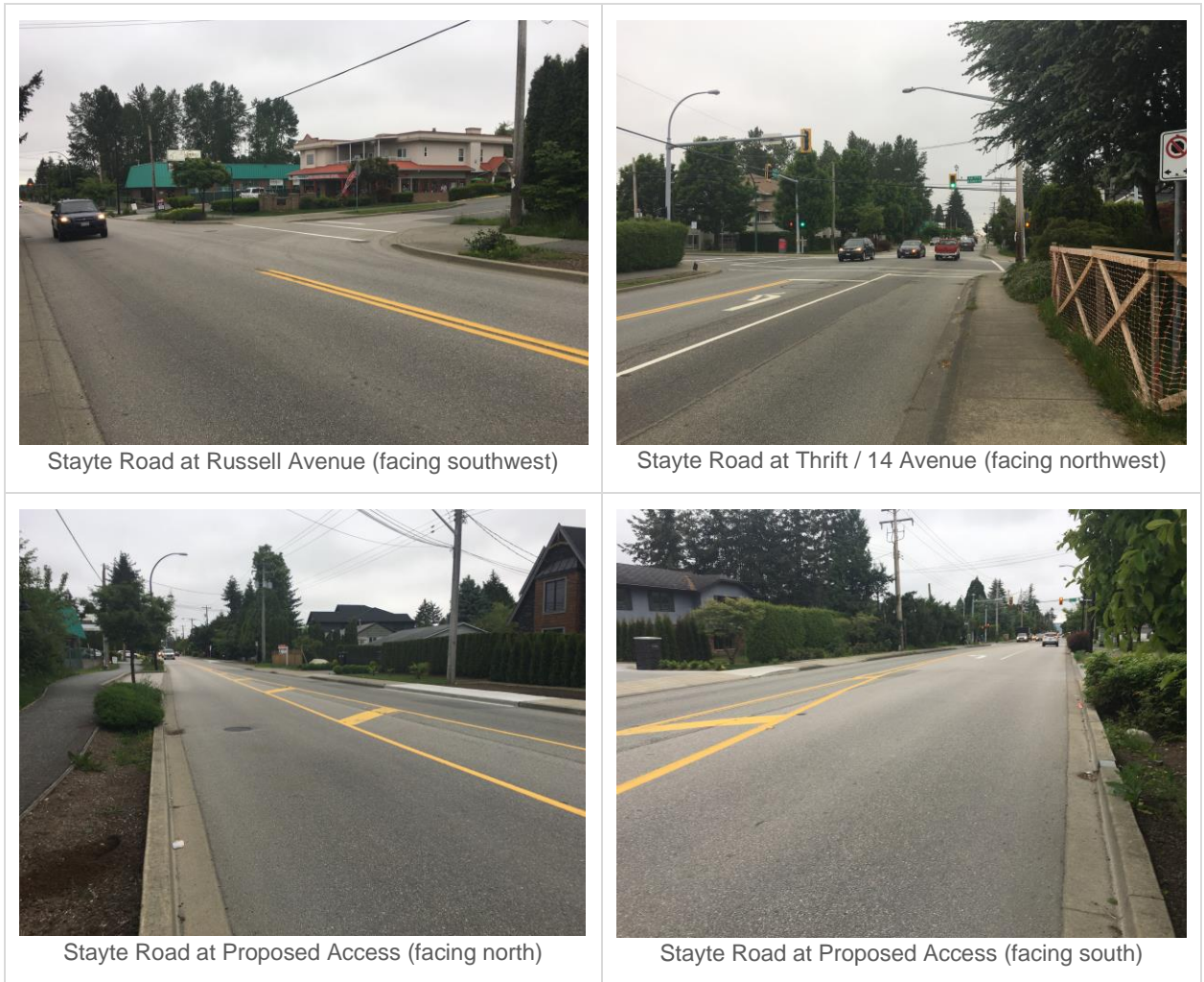
Figure 3 Site Visit Photographs
