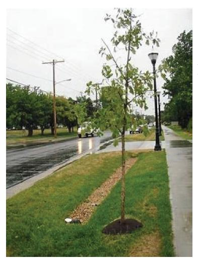
This illustrates an example of an easy way to maintain the system of infiltration through the use of a buried permeable pipe with a peak overflow to the storm system. This will help maintain a healthy water table.
