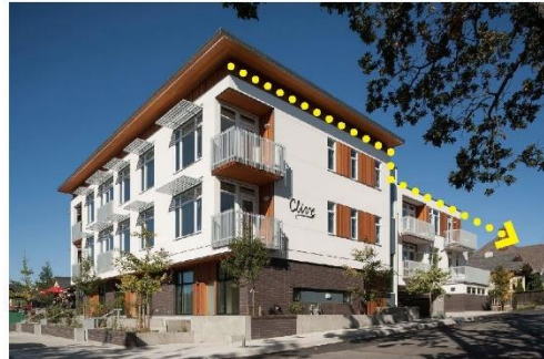
Guideline a and e: Addressing both street frontages and stepping down and back to create a smoother transition to the adjacent, lower density residential area
