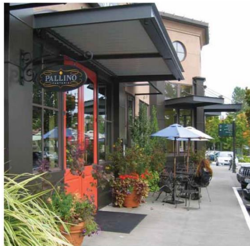
Guidelines c, d, g and k: Windows and colour variations along the front elevation, weather protection above the entrance level with the sidewalk, and projecting signage
