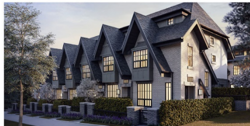
Guideline a and c: Materials, roof lines and front entrances create visual interest and soften transitions between multi-family development areas and single family areas
