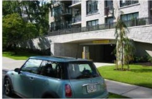
Guideline a: Parking entrances are designed to be discrete and softened by landscape
