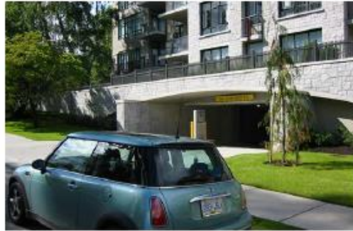
Guideline a: Parking entrances are designed to be discrete and softened by landscape
