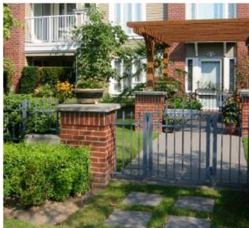
Guideline e: Landscaping elements establish a transition from public to private spaces
