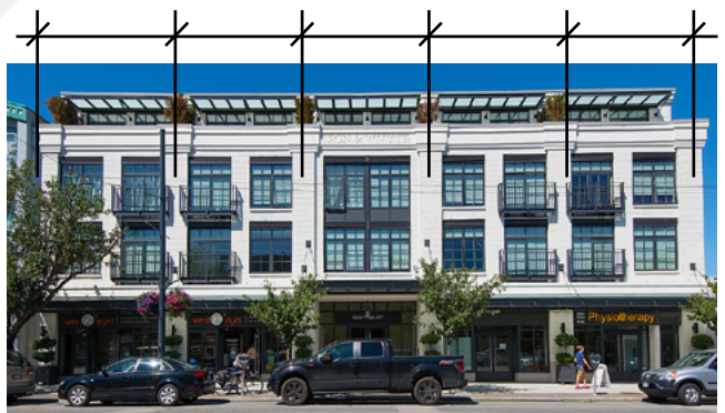
Guideline f: Facade articulation and narrow store fronts with entrances at regular intervals
