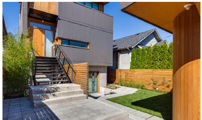
Guideline i: On-site parking using pervious materials
