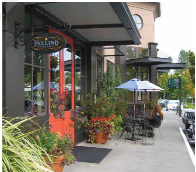
Guidelines c, d, g and k: Windows and colour variations along the front elevation, weather protection above the entrance level with the sidewalk, and projecting signage
