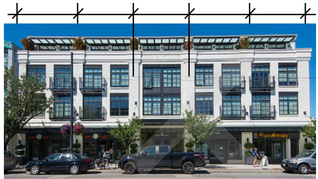
Guideline f: Facade articulation and narrow store fronts with entrances at regular intervals
