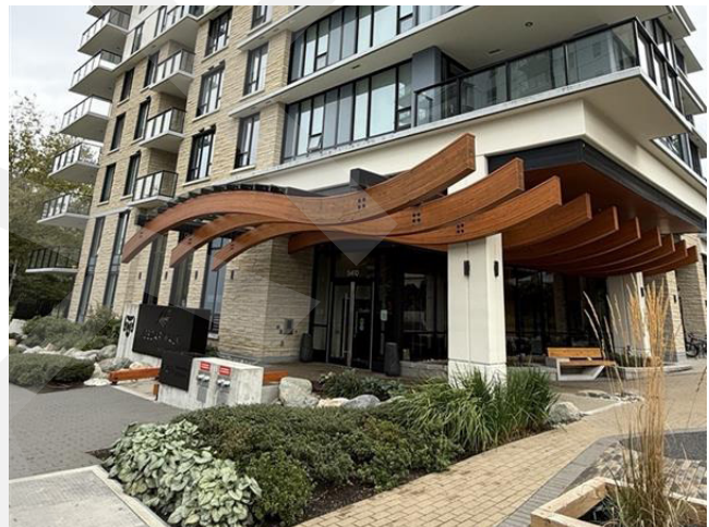
Guidelines d and e: Building entrances are level with the sidewalk and weather protected with architectural detailing along street frontages and walkways
