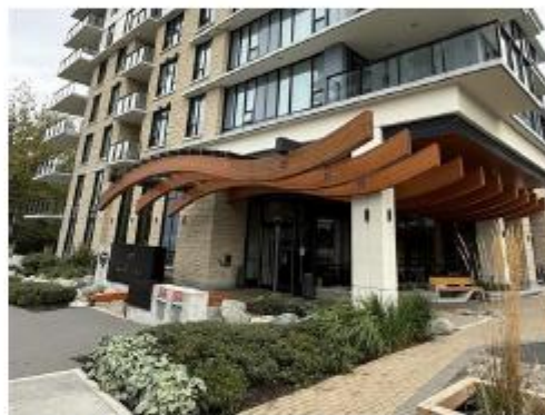
Guidelines d and e: Building entrances are level with the sidewalk and weather protected with architectural detailing along street frontages and walkways
