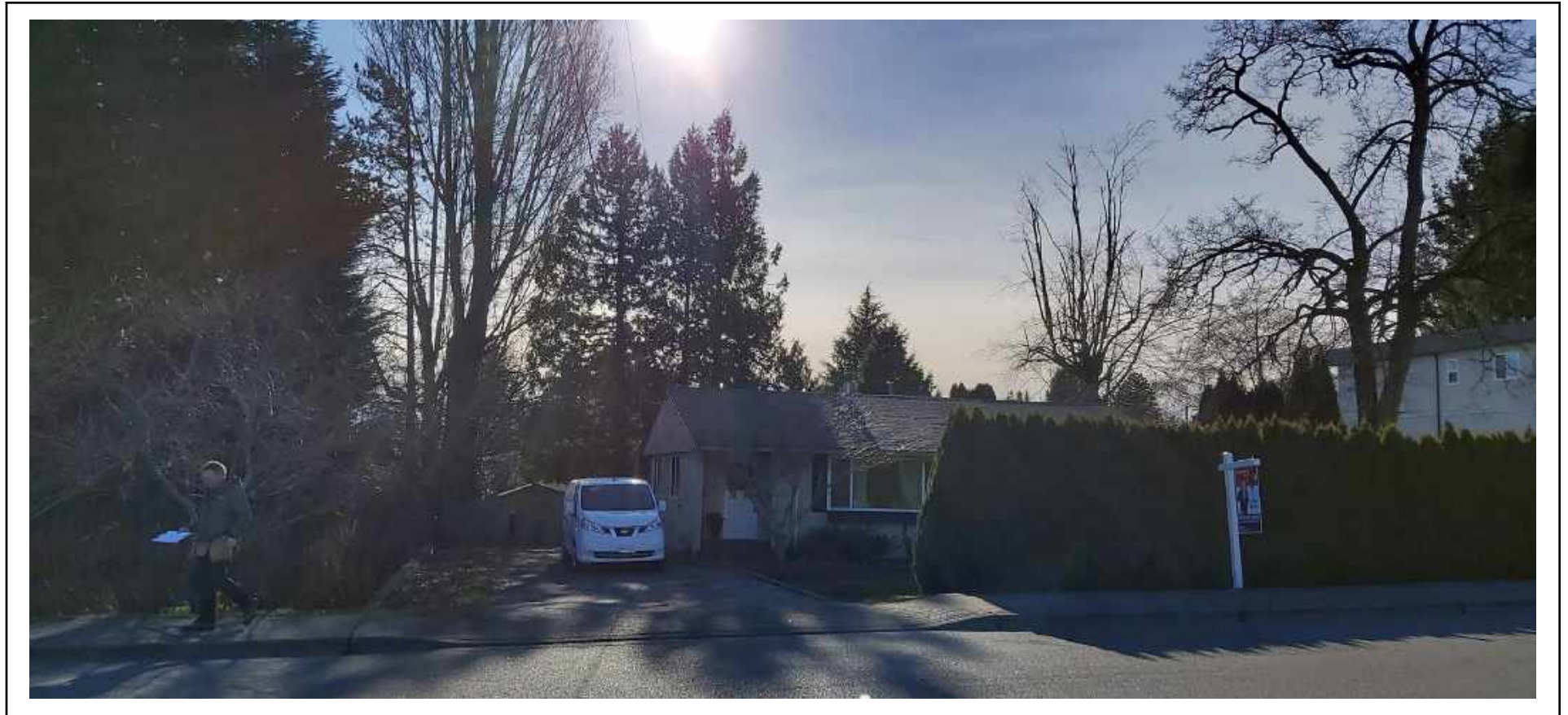
image of property from street at time of field data collection
