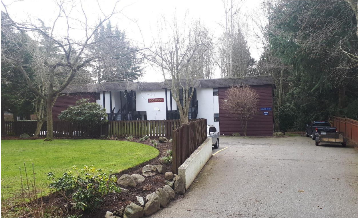
Photo 3: Looking south towards Building 1, one new parking space proposed in the location of the truck on the right hand side of the image.
