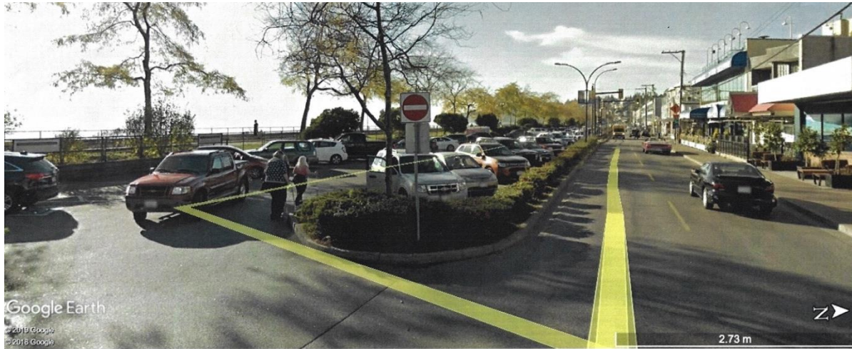
BEFORE: Marine Drive looking west along Marine Drive at Museum in West Beach
