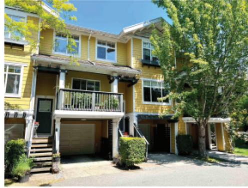
Guideline 22.8.4 (g), Garage Design and Placement.
