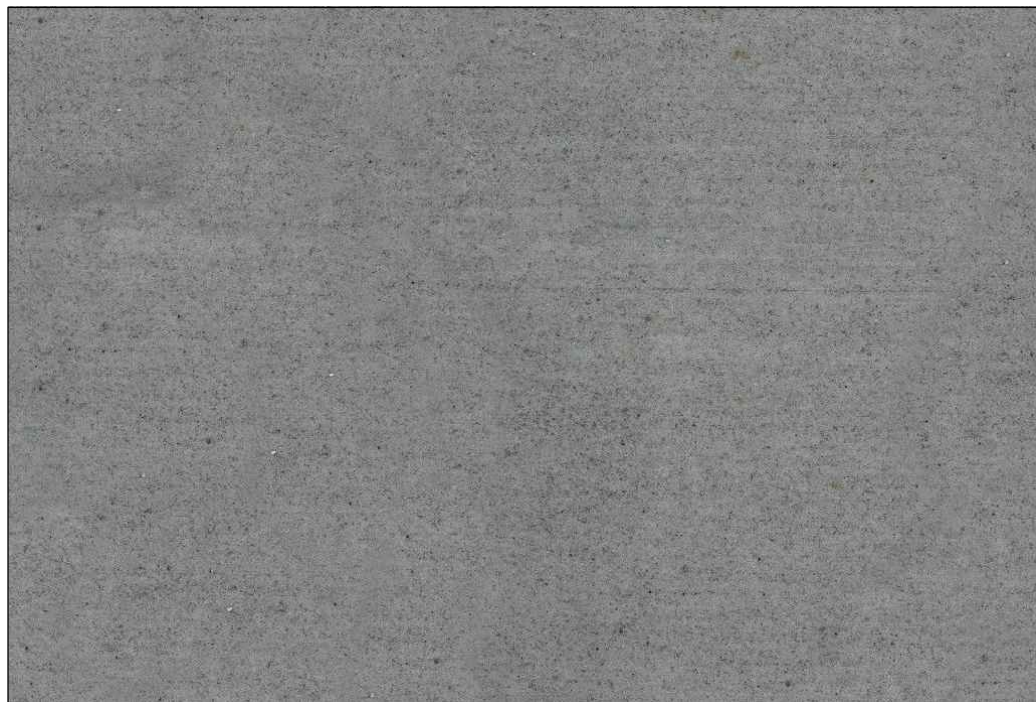
6 ARCHITECTURALLY FINISHED CONCRETE - LIGHT SAND BLAST
