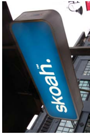
Unacceptable: Internally illuminated plastic face, back-lit "box" sign too thick and exposed electrical conduit to supply building.
