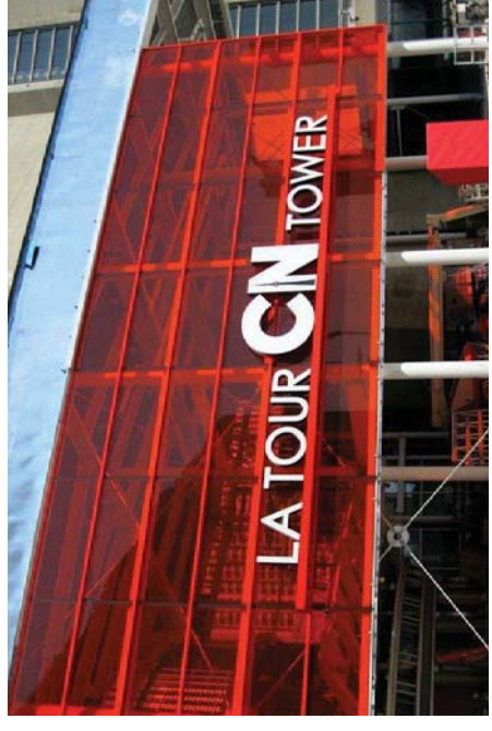
Sign well integrated with building glazed fascia
