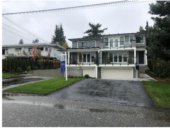
New Duplex - North side of Oxenham Avenue
