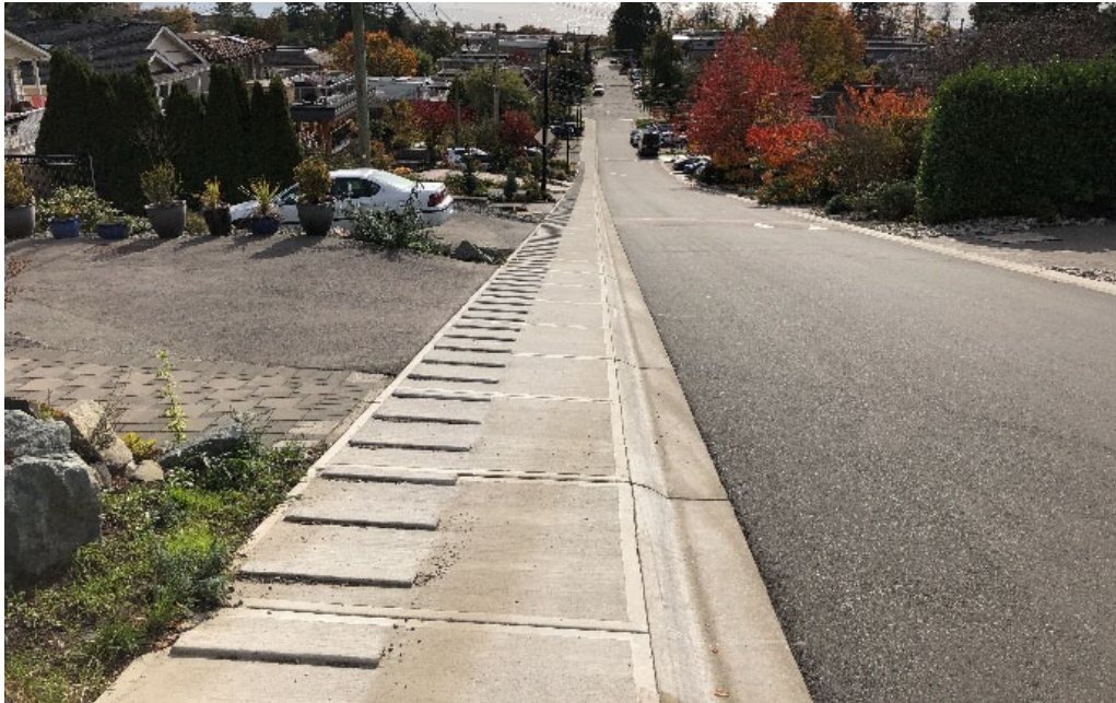
This street in White Rock is almost completely hard surfaced to provide vehicle parking on the City right of way.
