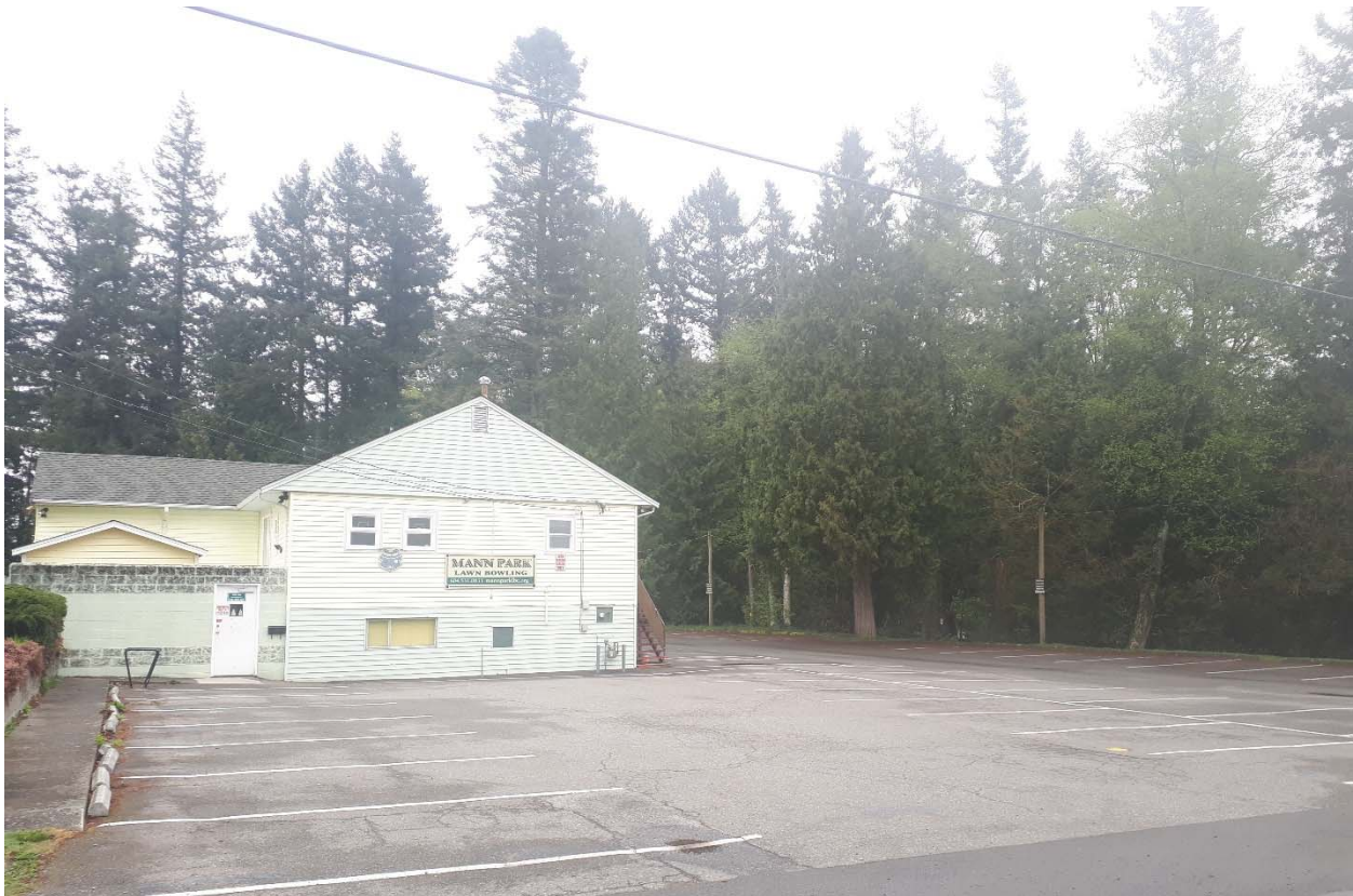
Figure 4: Parking lot servicing the subject property and the Tennis Club, note wooded lands south and east of the property
