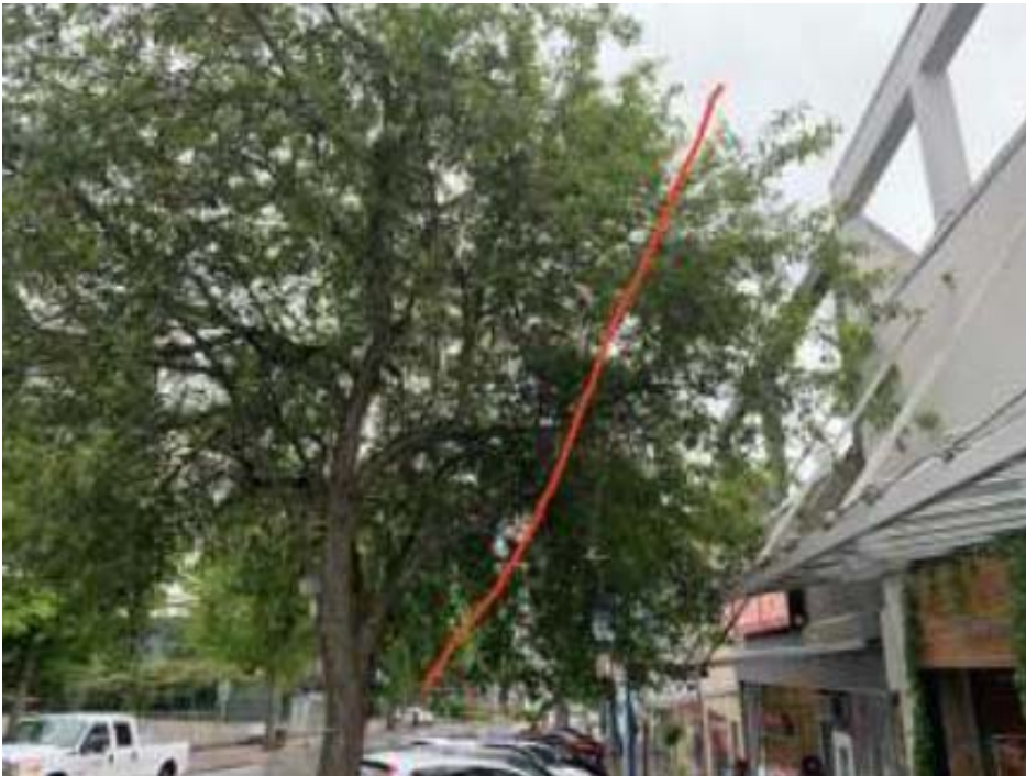
Figure 3: Building Clearance Issue – Johnston Road south of Prospect Avenue.
