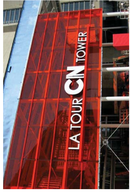
Sign well integrated with building glazed fascia
