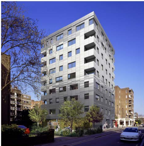
Case Study | Stadthaus, Murray Grove, London - Eight storeys of apartments featuring cross-laminated timber panels. TRADA Technology 2009.
