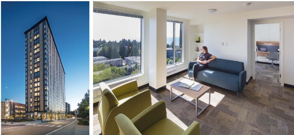
Seagate Structures, Brock Commons Construction Overview, Brock Commons, UBC
