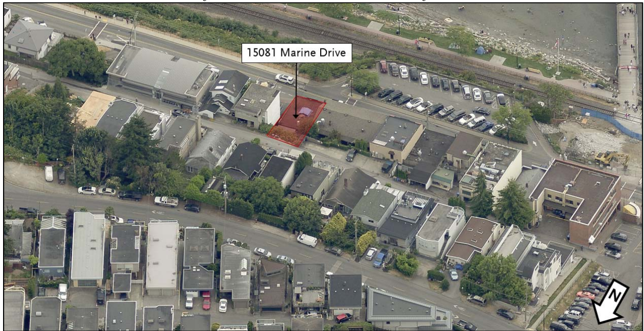
Aerial View of 15000-block Marine Drive from Northwest
