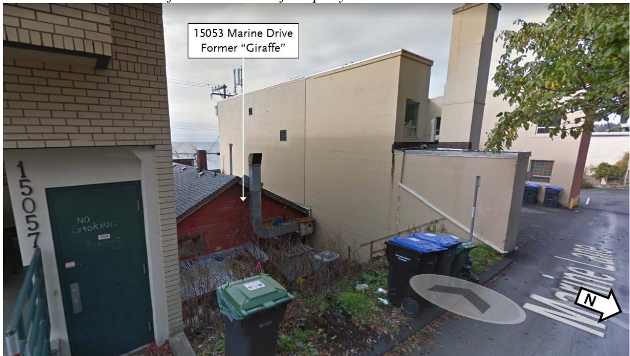
View from Rear Lane of Property at 15053 Marine Drive
