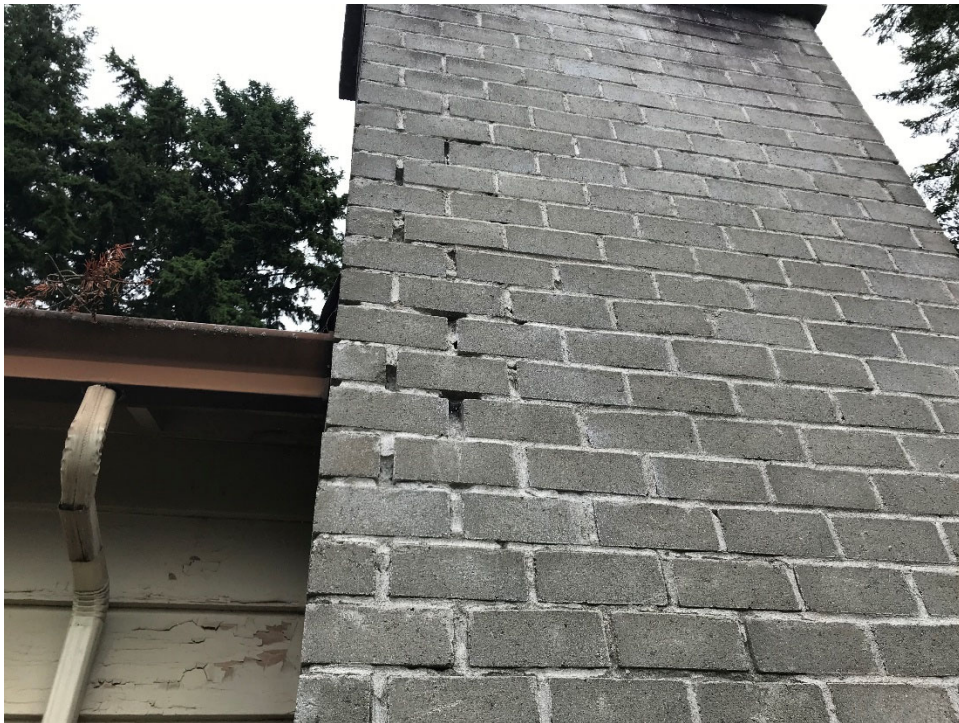
Grout Failure
