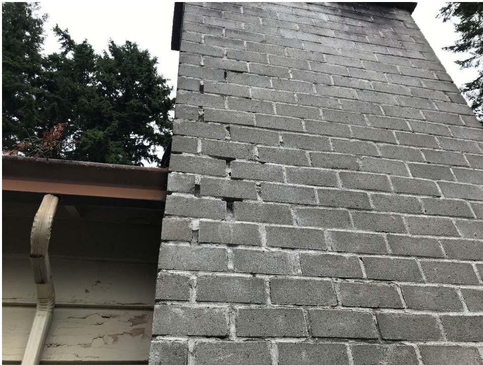
Grout Failure
