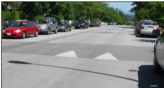
Example of a Speed Hump Treatment
