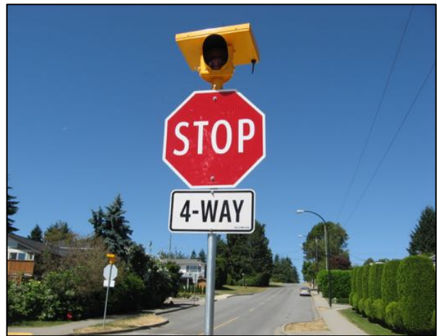
Flashing Beacon installation at Kent St / Roper Ave
