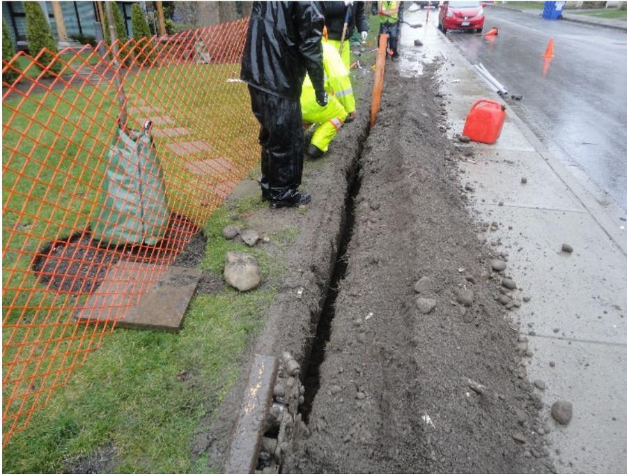
*This communication cable is located along the back of the sidewalk. Installing these cables in the roadway is much more expensive and may also conflict with other utilities.*
