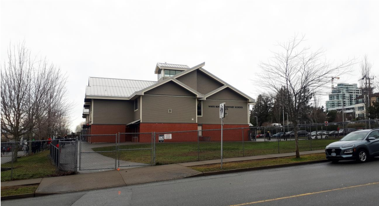
Photo 1: East Elevation of School
