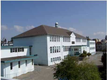
3 storey addition 1920's
