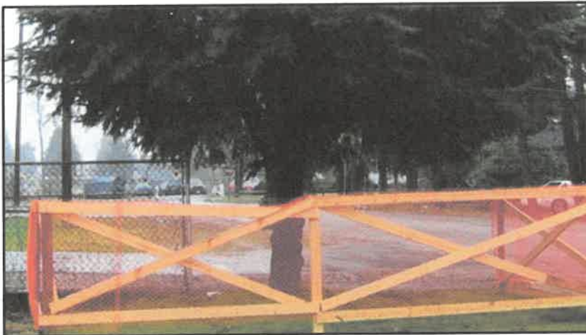
Tree Protection Barrier imagery taken from City of Surrey & City of Maple Ridge tree bylaws.
