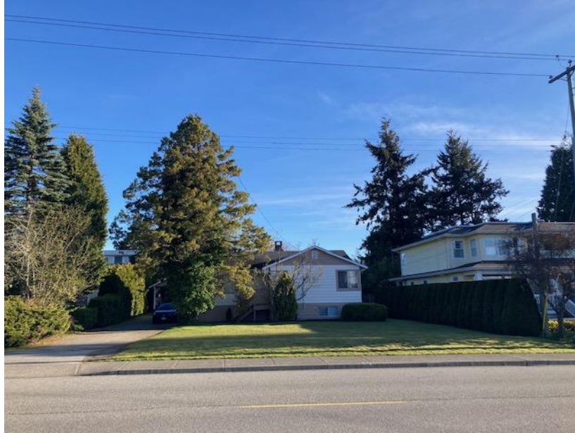
front view of subject property
