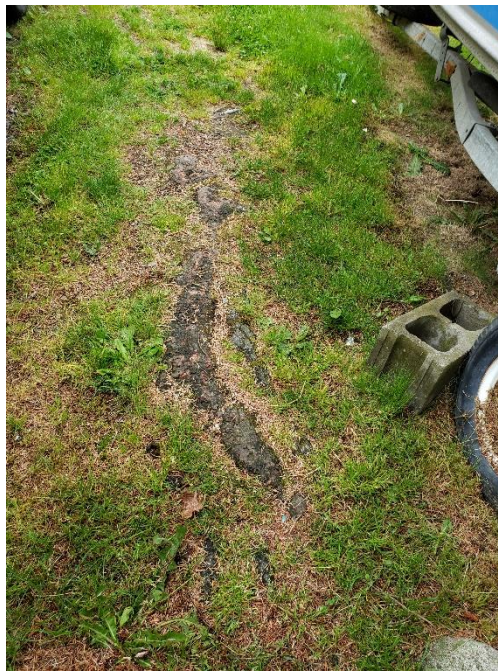
Surficial root getting damage from vehicle traffic
