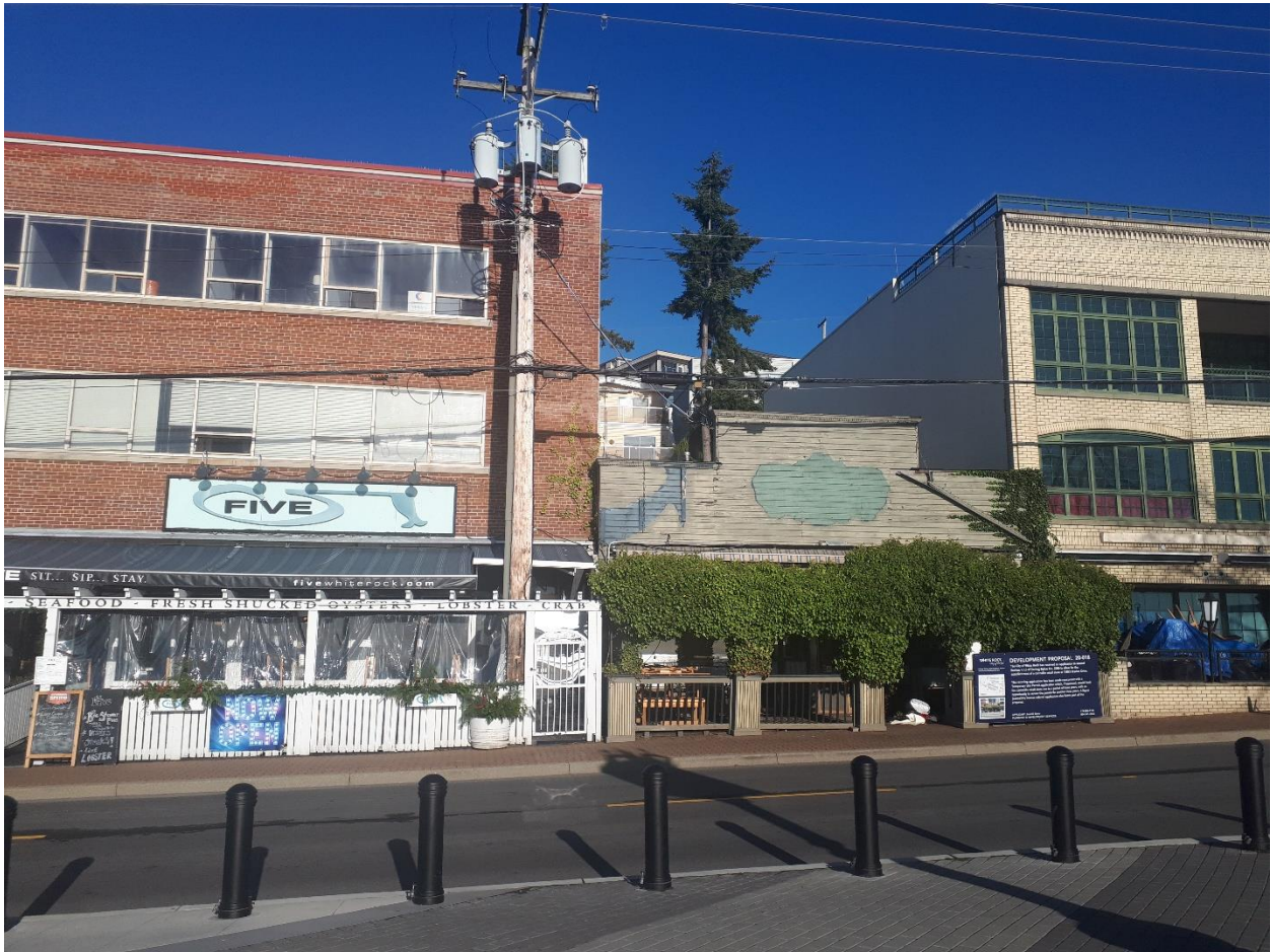
Photo 1: Front (Marine Drive) Facade
