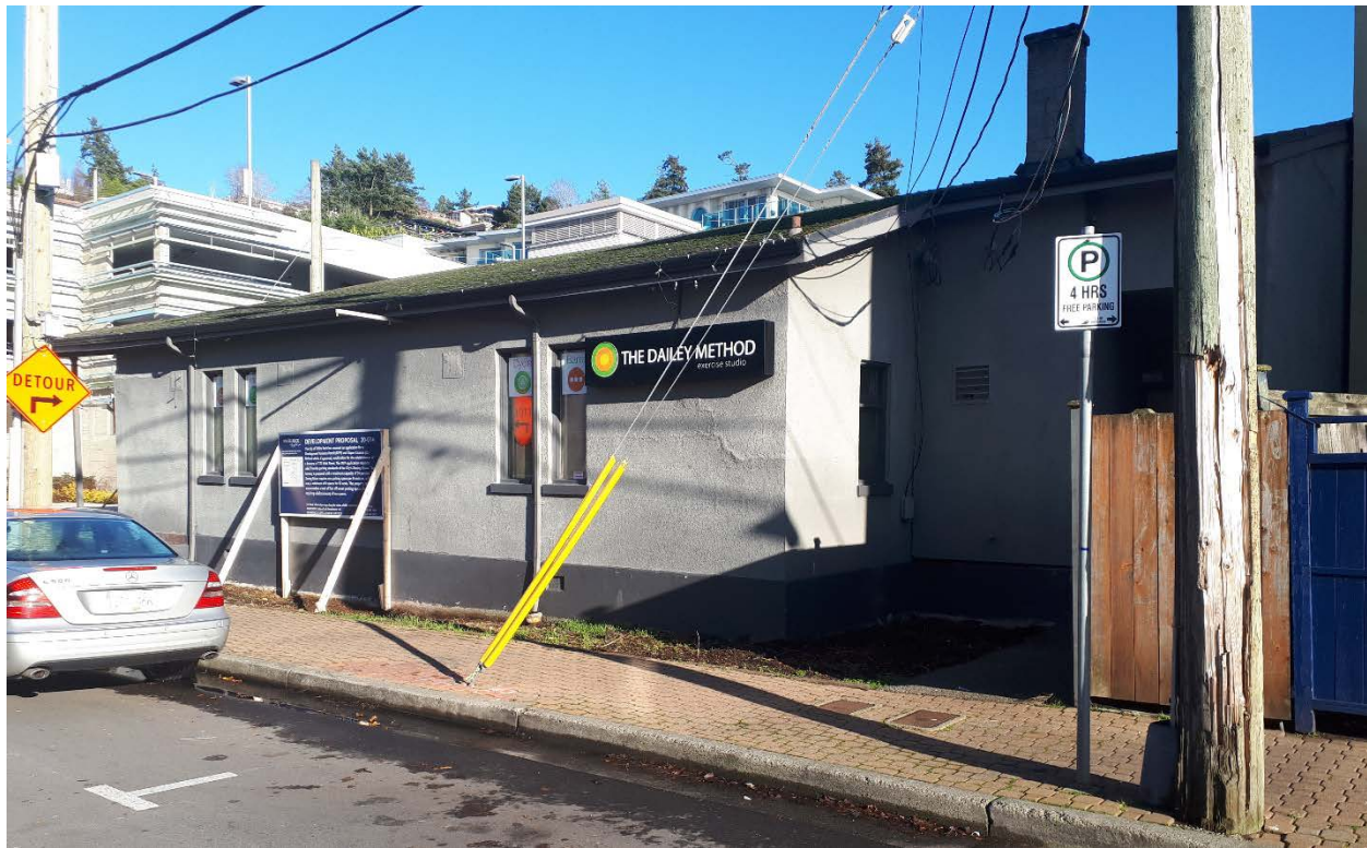
Photo 1: Subject Property (entrance on right side of image)
