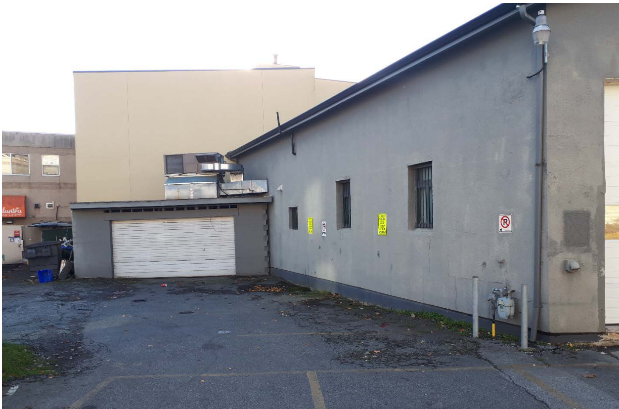
Photo 3: Rear (north-facing) elevation (painted lines to be adjusted to delineate four off-street parking spaces – will remove parking from City boulevard)
