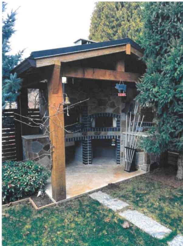
Figure 2: Existing Ancillary Barbeque Structure on the subject property
