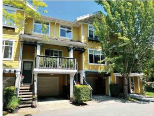
Guideline 22.8.4 (g), Garage Design and Placement.
